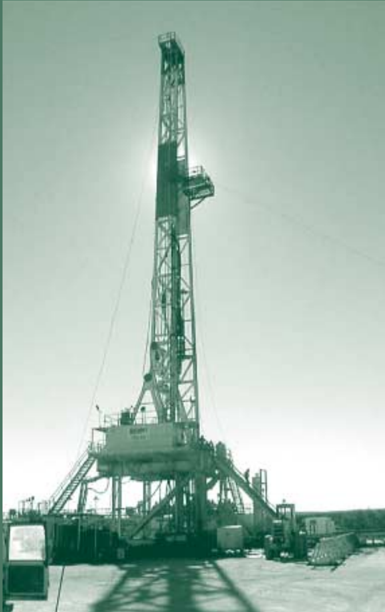
Drilling on the Jingemia Oil Field
